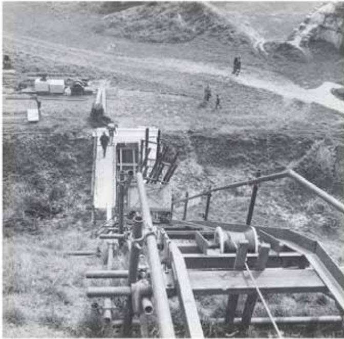
Fig.64. Arrangements for raising scaffolding and material to the Inner Ward in c.1959, HE Swindon, 6A19106. Reproduced with permission.
